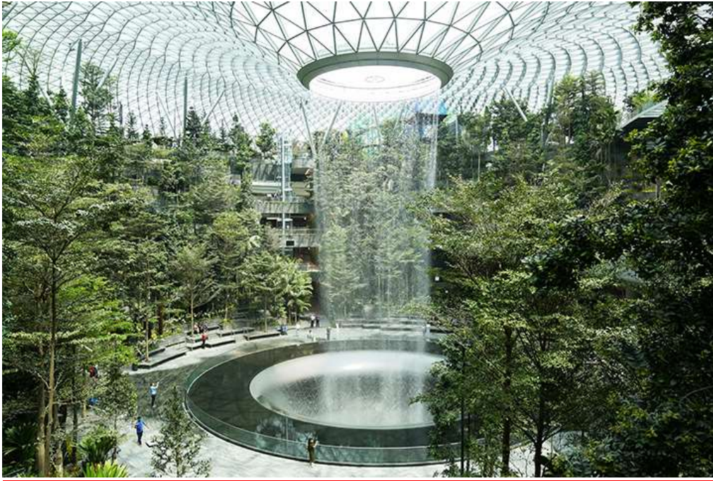
Singapore Airport has a funnel to collect rainwater
